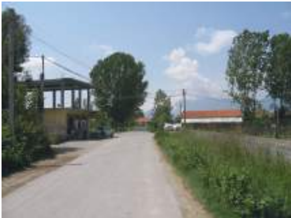
View of commune main road axis
