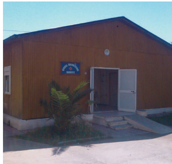
View of the health care center in Vau i Dejës City
