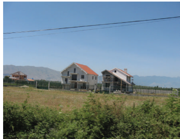
The residential developments along Shkoder-Koplik corridor
